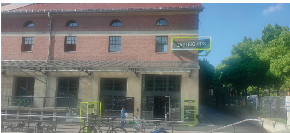
Figure 10. Outside view of Gasteig HP8
